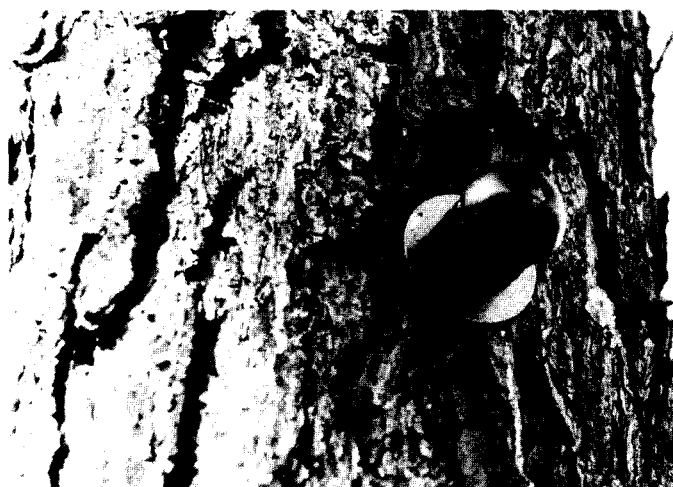
Figure 4—Lag screw installed in tree.
