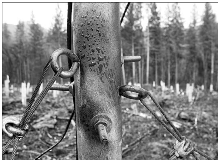
Figure 3. Guy wire attachment.
