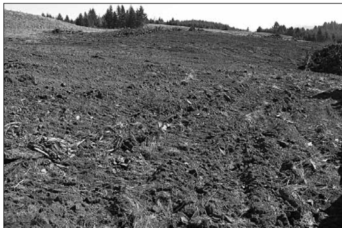
Figure 1. Clearing an area previously under trees.
