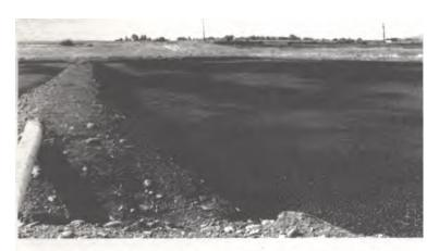
Figure 6. Sludge in drying beds following digestion. Vernon Thorpe Water Quality Control Plant, City of Medford.
